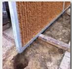
The topside of the panel is marked with a sticker (with arrow) at one side of the panel. Place the backside of the panel (with bolts / rivits in corners) to the side of the posts without drilled mounting holes. In this way there won't be a gap between postflange (mounting side) and panel.
